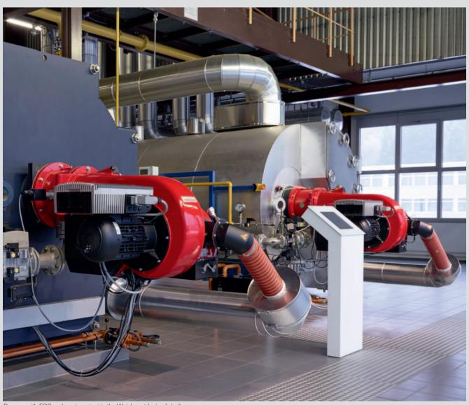
Burners with FGR on long-term test in the Weishaupt factory's boiler room
