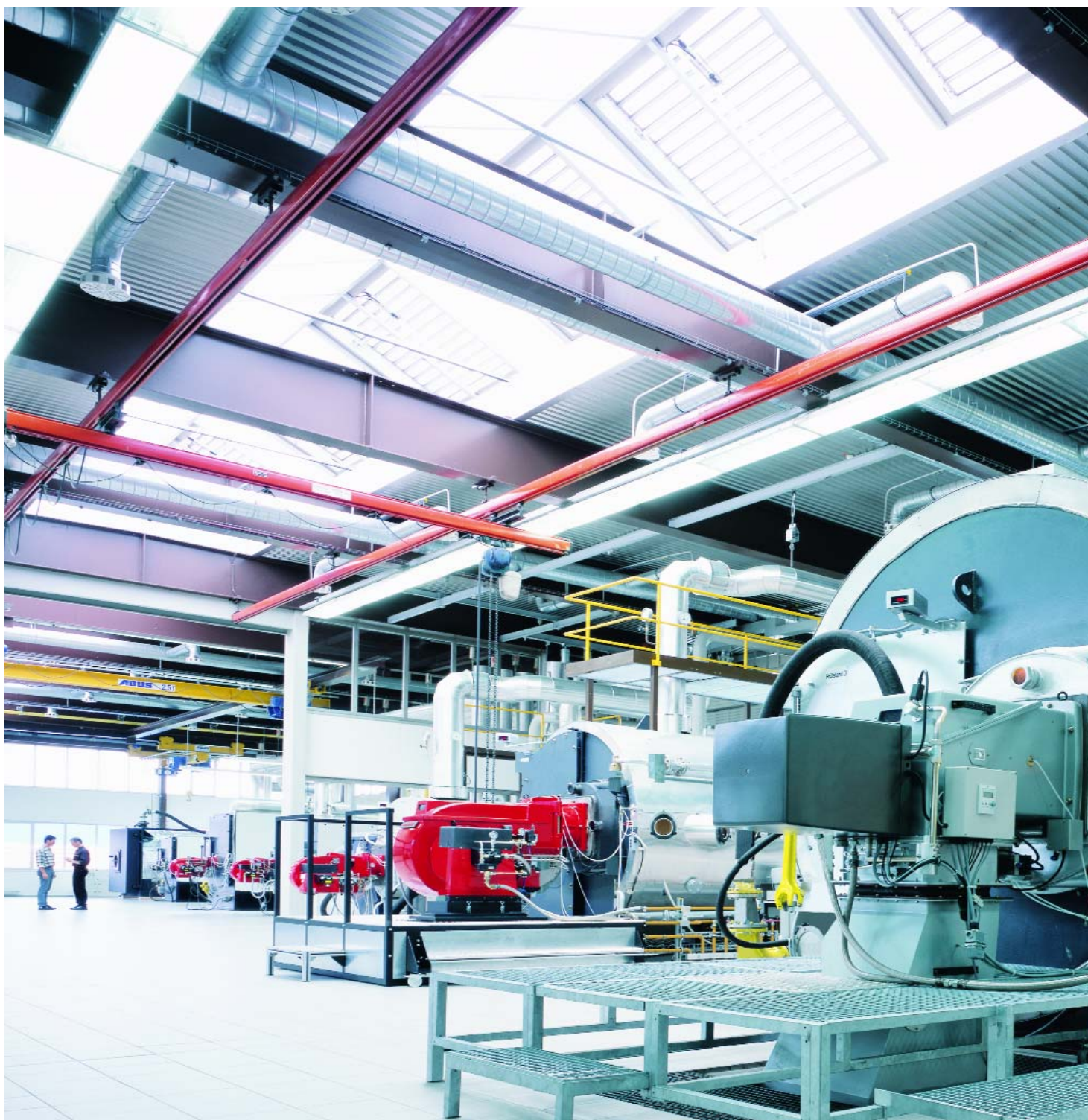
Test beds at the Weishaupt Research and Development Centre
